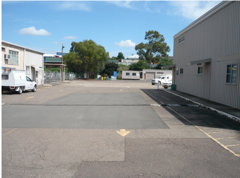
Plate No. 5: View of new bitumen indicating where the UST was removed
