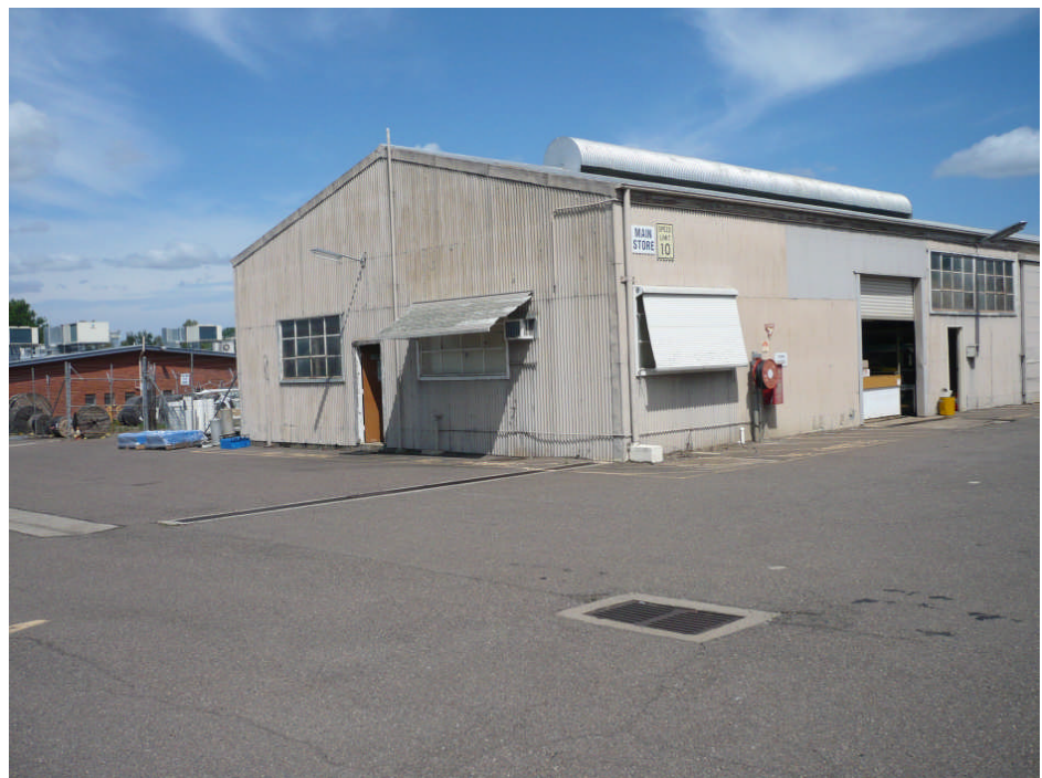
Plate No. 6: Building on site used for storage and maintenance purposes.
